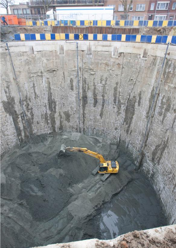
07 Excavations of a storm basin by the earthworks company De Meuter in Brussels. The Ypresian geological layer, a cohesive clay, is laid bare, and is one of the resources that BC materials uses to make building materials. (Photo: De Meuter)
