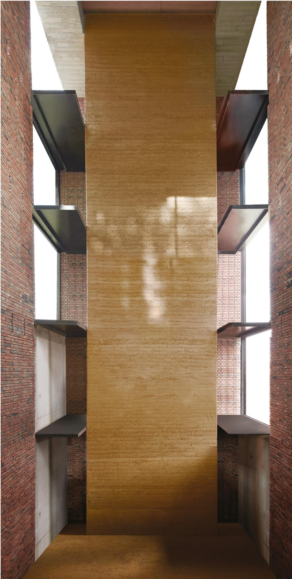
12 WALL: A 15-metre-high rammed earth wall by BC materials and Het Leemniscaat for AST77 architects. The rammed earth mixture was made from soil from the site with the addition of sands and gravels. (Photo: Steven Massart)
